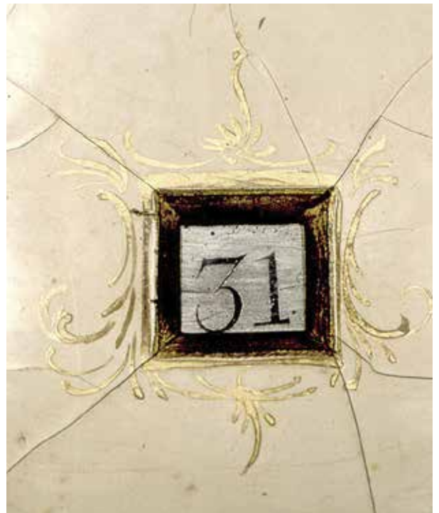
Figure 8 (above left). Repoussé brass spandrels riveted to the iron dial sheet. Photograph J Betts.
