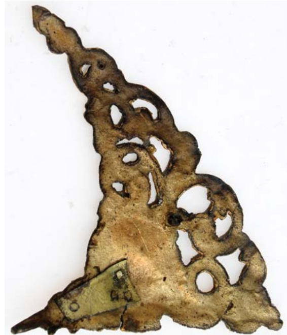
9. Rear of the arch spandrels. The one on the right has been repaired using a riveted strap. The one on the left has been cast using a similarly repaired original as a pattern.
