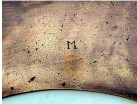
Fig. 2. M casting mark on the chapter ring of an 8-day longcase dial signed for Richard Monkland, Worcester, about 1740. The dial was probably engraved in Bristol.
