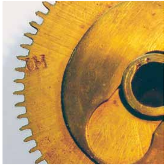
Fig. 7. IM mark on the hour wheel of an 8-day clock by Stephen Wilmshurst, Odiham, about 1720. (Photo: M. Forrester)
