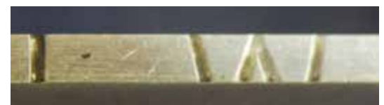
Figure 10. The bottom edges of the plates filed with 'IW' for ease of assembly.
