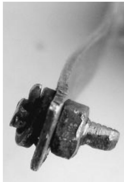
5 A crude replacement rack tail.
