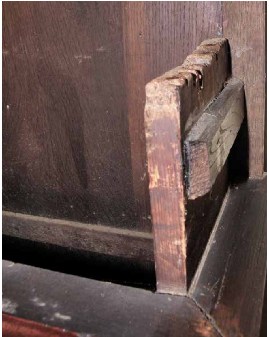
Figure 13. The cheeks on which the seatboard sits have never been altered.
